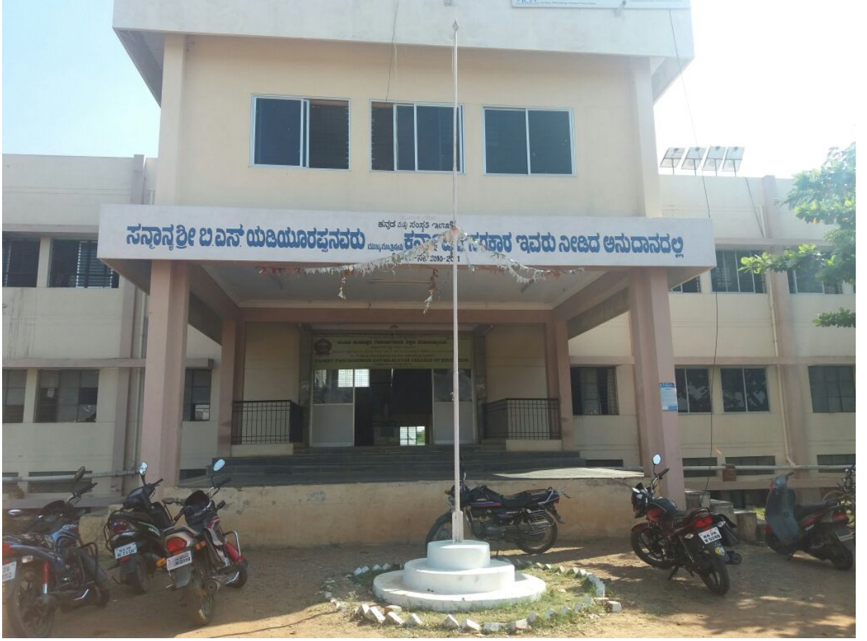
Rear view of the building
